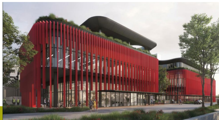
EG: NEXT DC S4 DATA CENTRE, HORSLEY PARK 232MW
