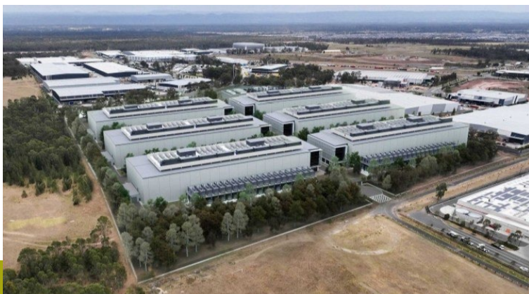
EG: CDC DATA CENTRE MARSDEN PARK, 504MW CAPACITY
